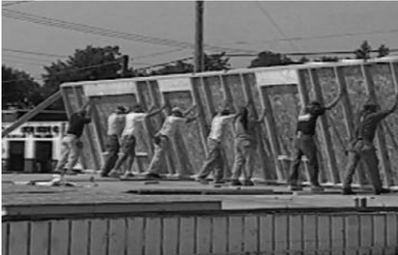
Volunteers raise the first wall in August!
